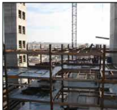
Construction of the East Tower, funded by the 2007 Bond.
